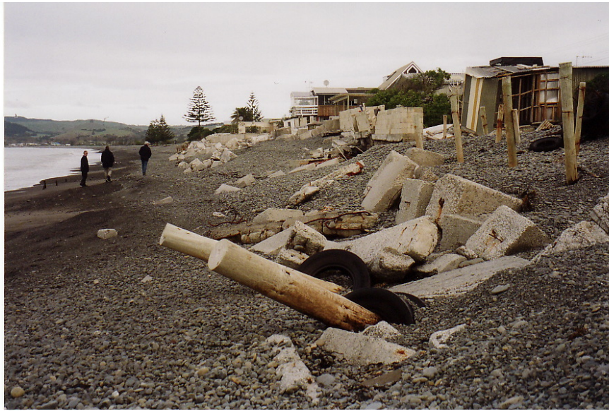
Figure 1-9: Erosion and property damage in the community of South Haumoana, in part attributed to the subsidence of this shore during the 1931 earthquake, but with its sediment budget “in the red” being the primary cause. [Photo, 2005]
